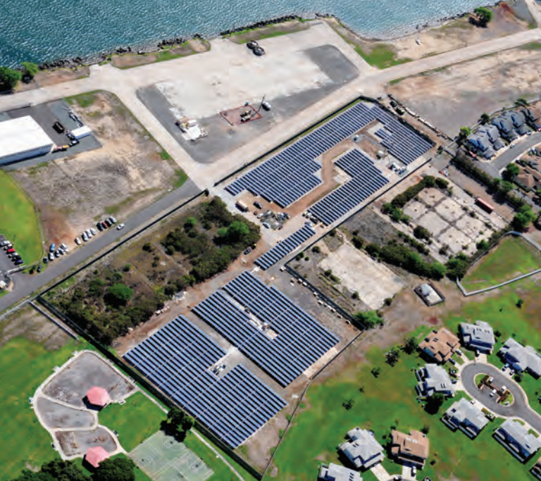
Pearl City Peninsula solar farm built by Forest City in 2012
